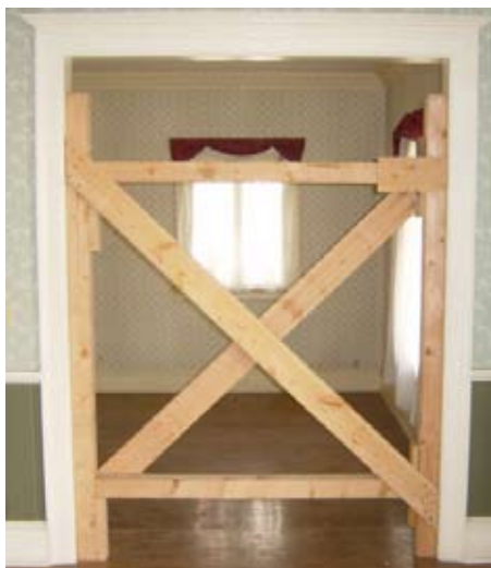
Figure 6:39 Horizontal Shore
