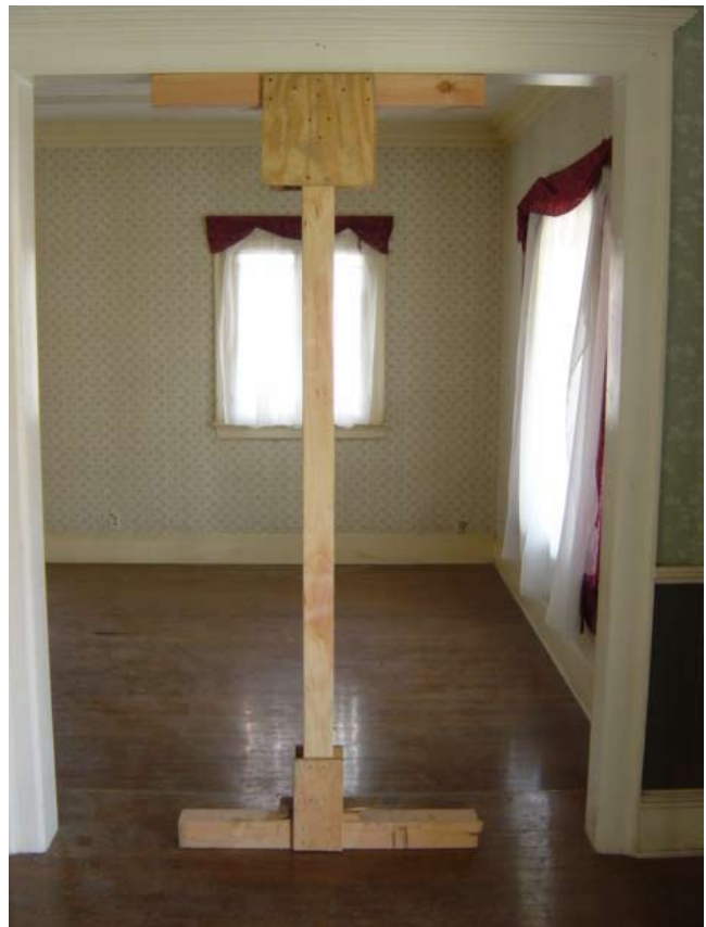
Figure 6:34 Timber Spot Shore
