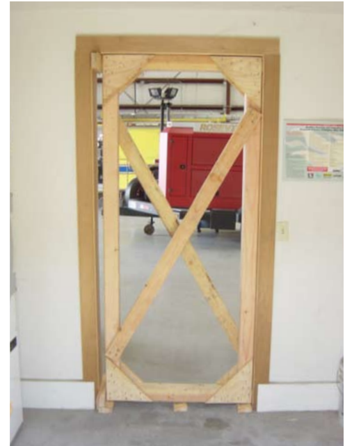
Figure 6:21 Window and Door Shore
