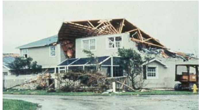
Figure 6:3 Light-Frame Collapse
