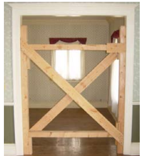
Figure 6:19 Horizontal Shore
