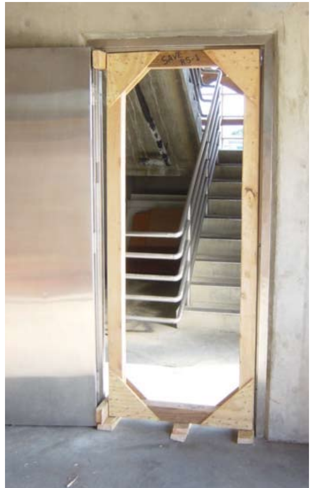
Figure 6:41 Window and Door Shore
